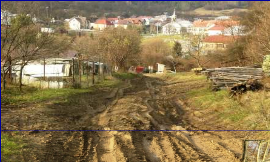
Erosion on roads
